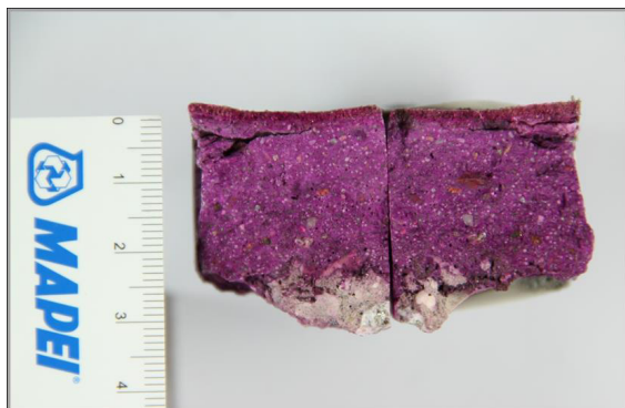
FIG. 20.8 - SAMPLE TAKEN FROM THE STRUCTURE AND ANALYSED WITH PHENOLPHTHALEIN: THE TOTAL ABSENCE OF CARBONATION IN THE CONCRETE THICKNESS CAN BE SEEN
